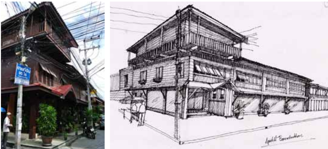
Figure 20. The Sathukarn House on Krasaesin Road.
