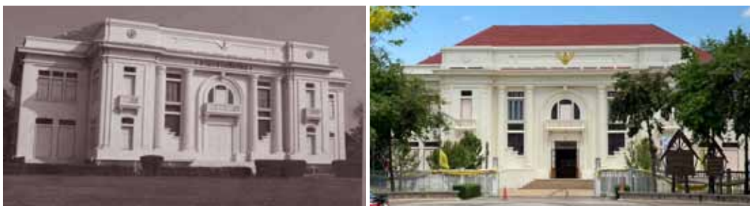
Figure 7. The front façade. During renovation, a ramp was added to both wings of the building, although the building retains its unique character. Left: (Siam 2015), right: photo by the author.
