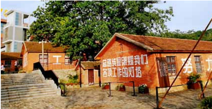
Figure 12. Restoration of mining factory and residential area. Source: the author.
