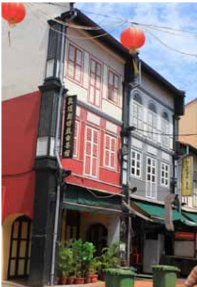
Figure 10. Shophouses in Clarke Quay and Boat Quay. Source: Author, 2019.
