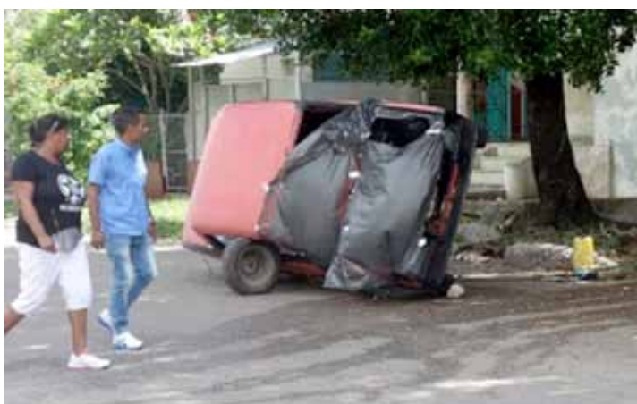
Figure 4. Creative private repair works in progress as spare car parts needed to be sourced, in the non-touristic neighborhood away from Havana old city centre.
