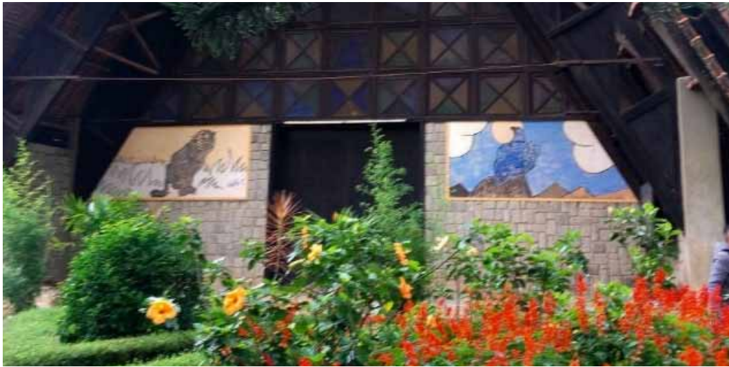
Figure 12. An outside wall of the CamLy Parish Church, Dalat, Vietnam.
