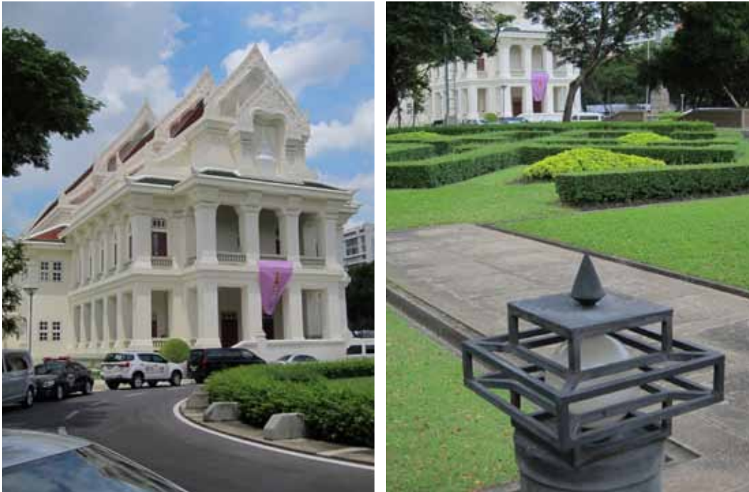
Figure 1. Two views of the Maha Chulalongkorn Building on campus – A. Kinear.
