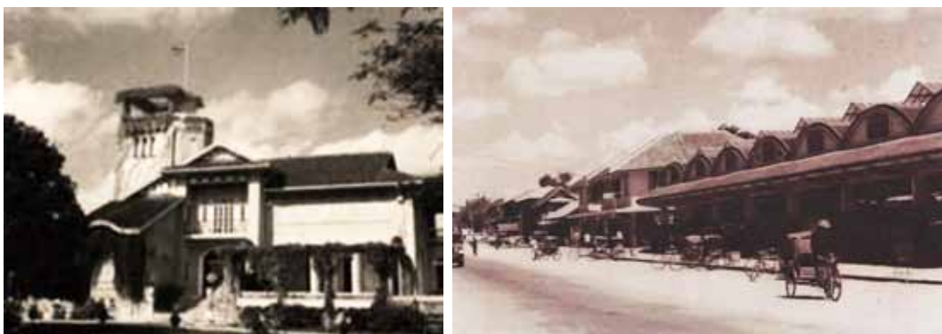
Figure 6. Piam Suk Building, Klai Kangwon Palace, left and the Chatchai Market, right.
