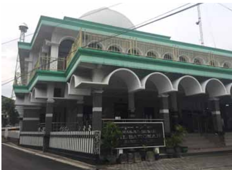
Figure 7. Al Barokah mosque or has been known as Masjid Bambu Runcing. Source: Private documentation, 2019.
